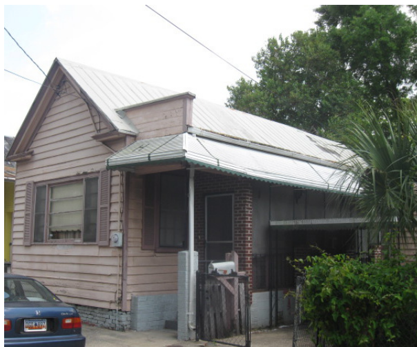
Historic Charleston Foundation (HCF) has operated a revolving fund since 1957. HCF used its fund to restore the facade and piazza of this small "Freedman's Cottage" in 2012. Photos courtesy HCF.
