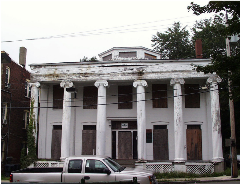
Alvah Kittredge House in Roxbury
