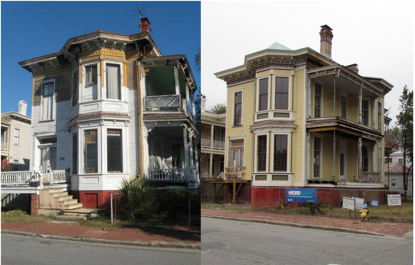
Before and during rehab pictures of the P.J. O'Connor House
