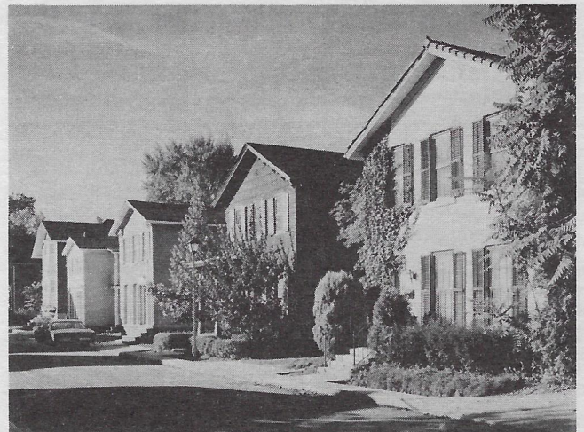
Greenwood Street, Third Ward Historic District, Rochester. The two houses in the foreground were purchased and resold through the revolving fund as part of a Landmark Society demonstration project.
