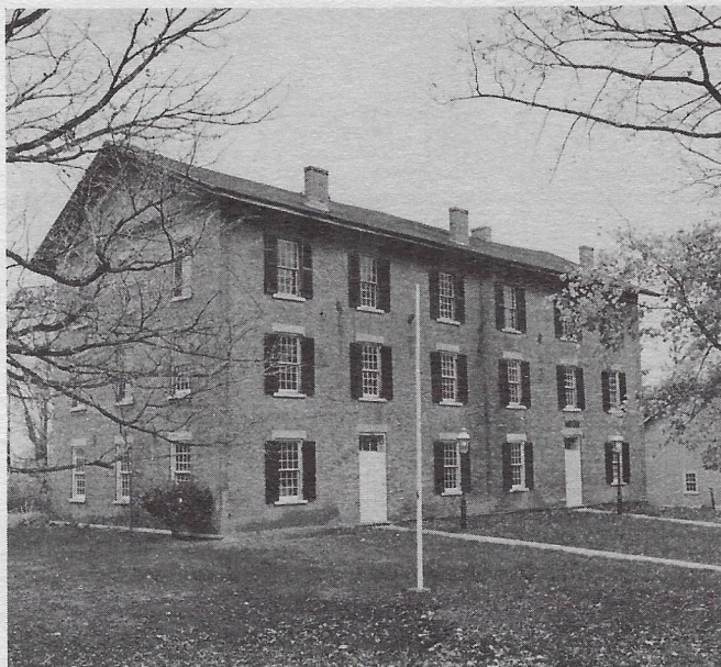
East Bloomfield Academy, East Bloomfield, New York. This important building was saved from demolition and adapted for use as a museum and community center by the local historical society. A four-year loan from the revolving fund helped pay for emergency repairs.
