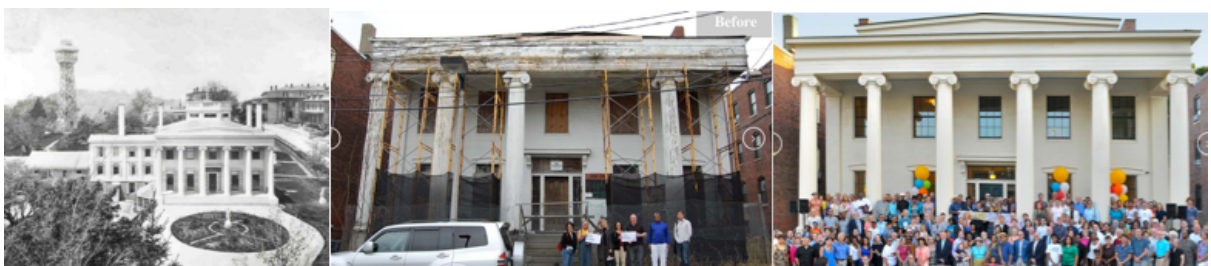
Figure 15-HBI's Alvah Kittredge House, Roxbury, MA-Historic Image, Before and After restoration-Images courtesy of HBI
