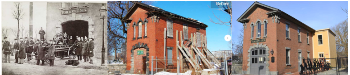
Figure 16-HBI's Eustis Street Fire House, Roxbury, MA--Historic Image, Before and After-Images courtesy of HBI
